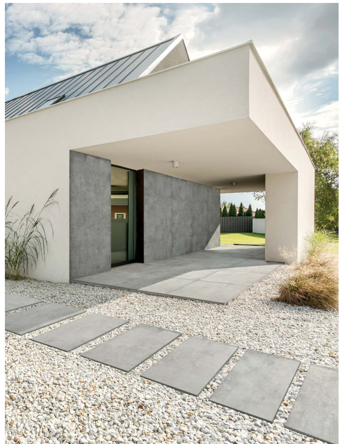
Example of the dry installation on the gravel.
